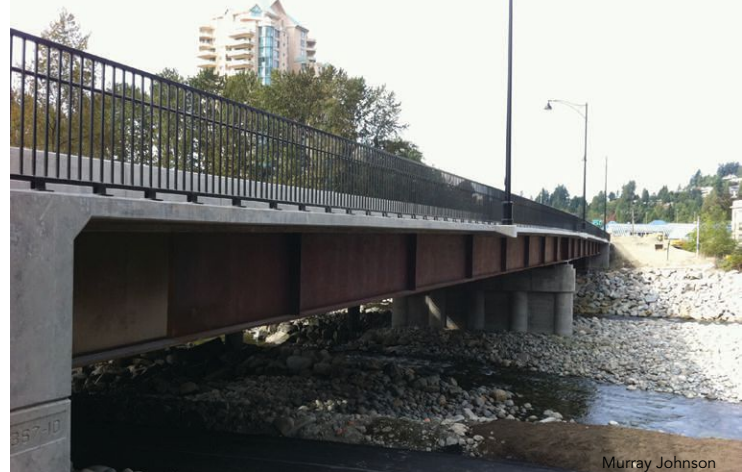
▲ The completed New Capilano River Bridge.
