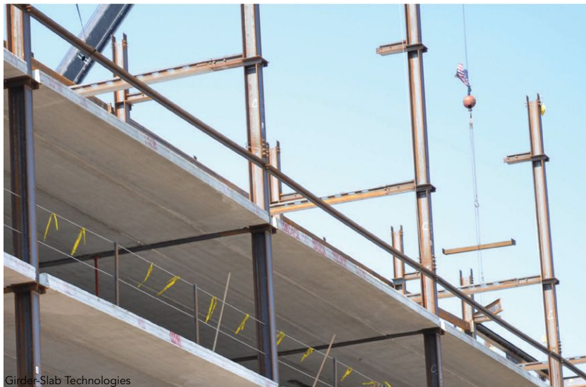
▲ Figure 5: Tree columns in place.
